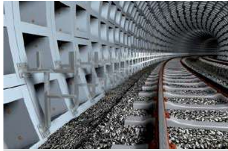
Installations in tunnels
