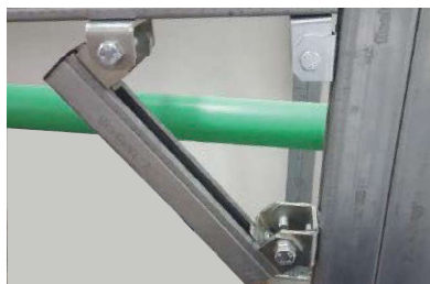
Height adjustable pipe installation
