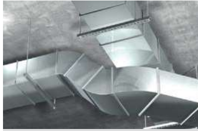
Repair of damaged hot-dip galvanised areas
