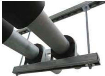
Suspended pipe support
