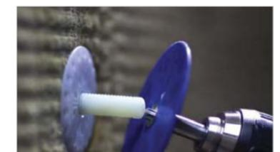
The most universal fastener – for all substrates (ABCDE), all types of insulation material and thickness, either countersunk or surface fixed, backed by European Technical Approval.
