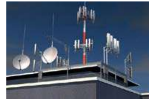
Antenna and masts
