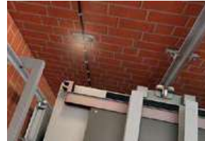
Elevator guide rails
